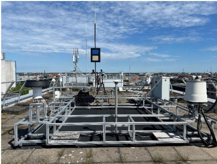
Sky scanner at the rooftop
